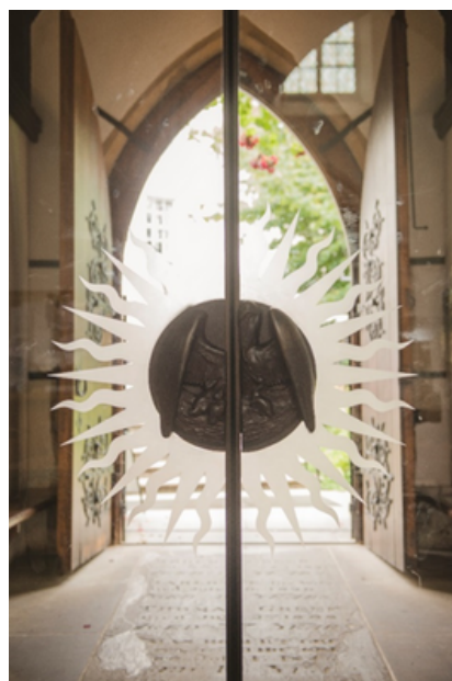
New automatic glass door with bronze pelican handles installed as part of the 2020 'Millennium Project' to improve disabled access to the church.
